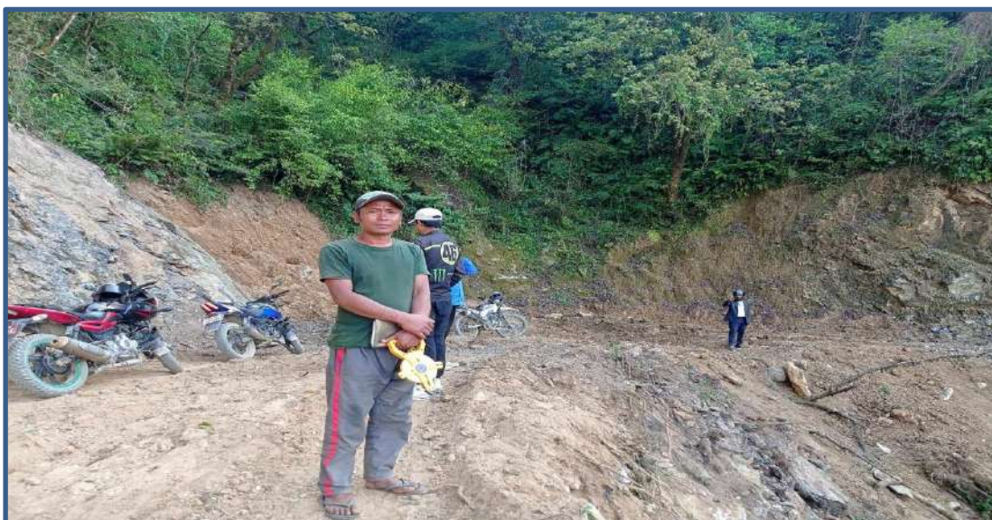
Track Joining Point (Sigdi-Tangram Road Section)
