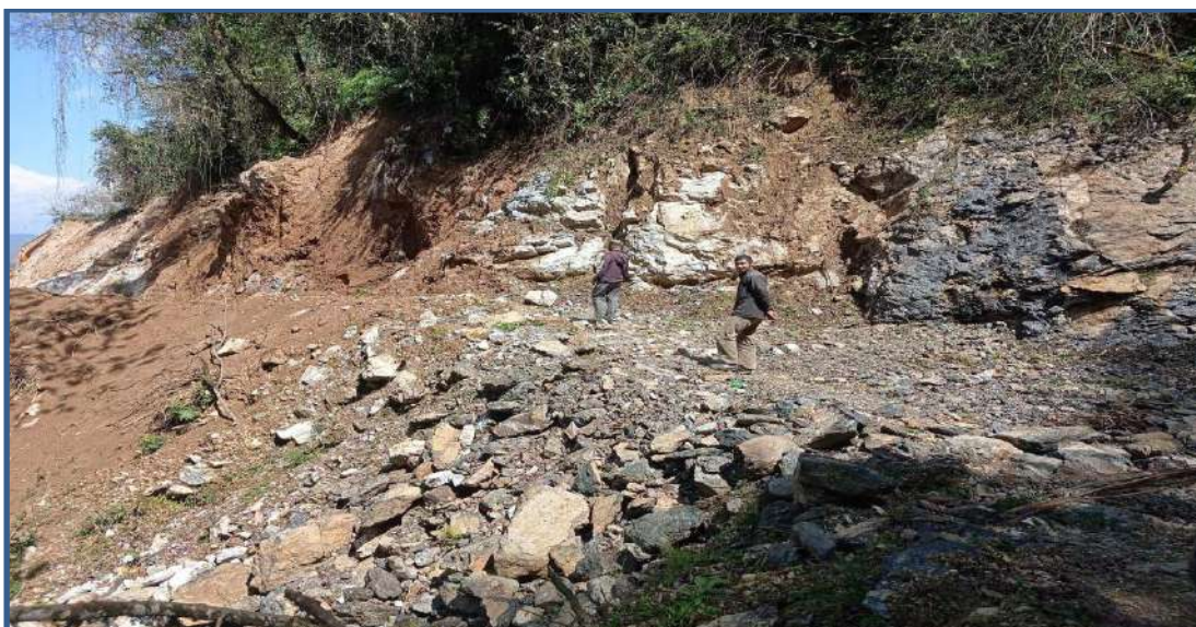
Track Joining Point (Sigdi-Tangram Road Section)
