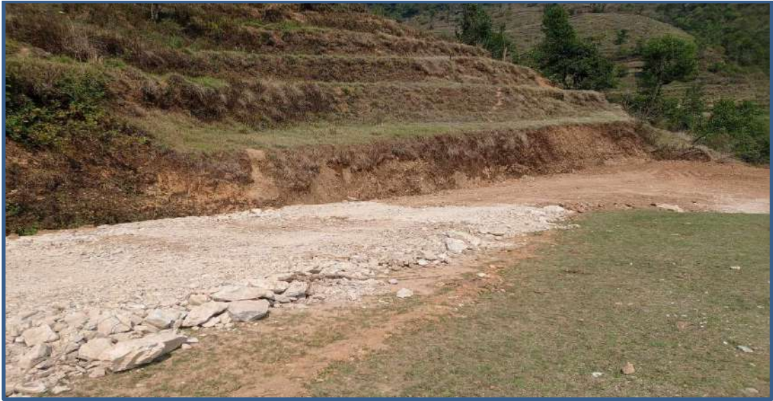
Gravel laying at sukhaura road section
