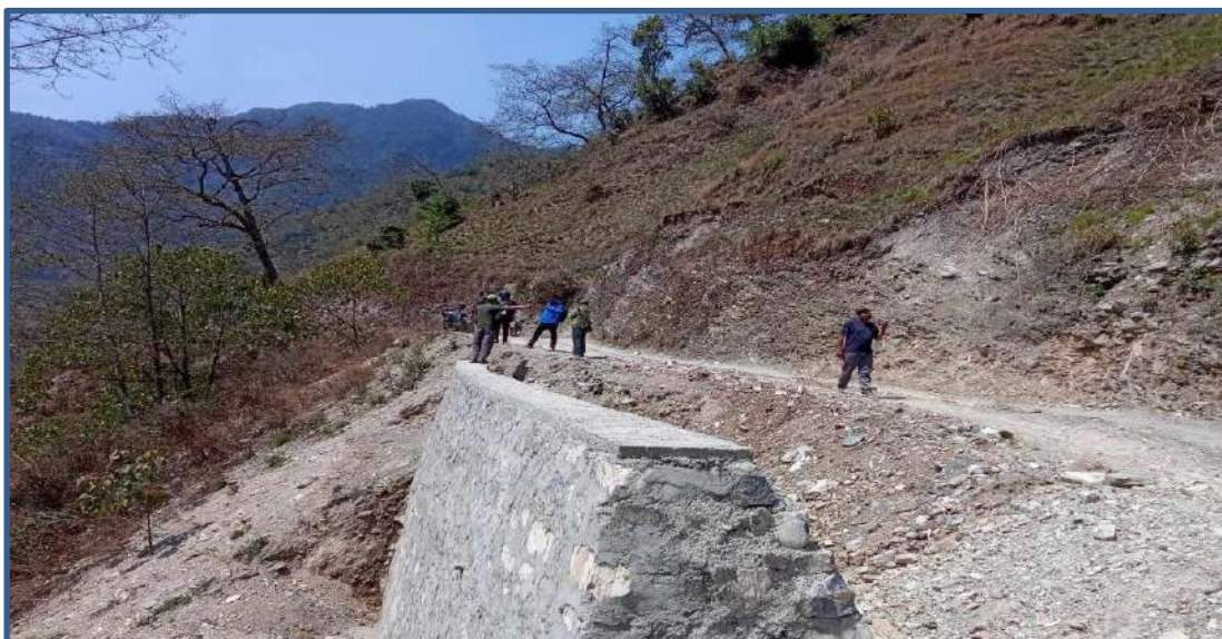
Site Inspection by Rural Municipality Officials (Jhule-Lugrung Road section)
