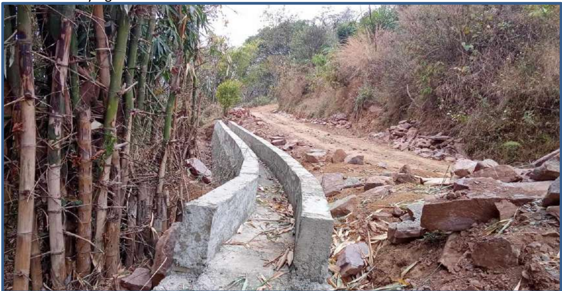
kudahara irrigation drain along with road
