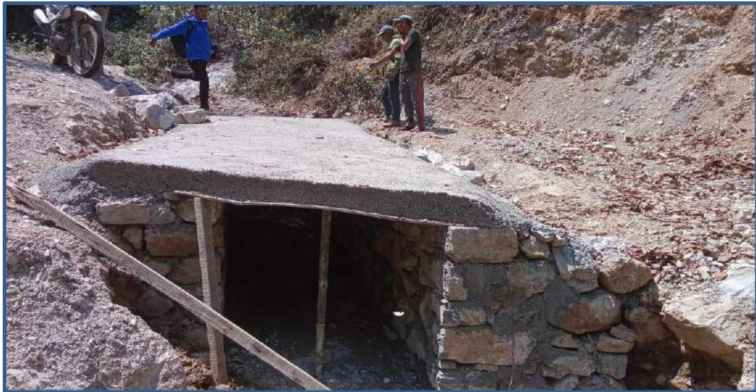
Cross-Drain Near to Timureghat
