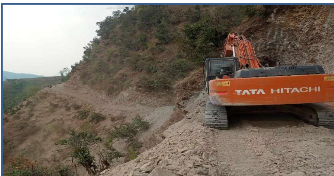
Road Cutting at Daduwa-Thaple Difficult Section
