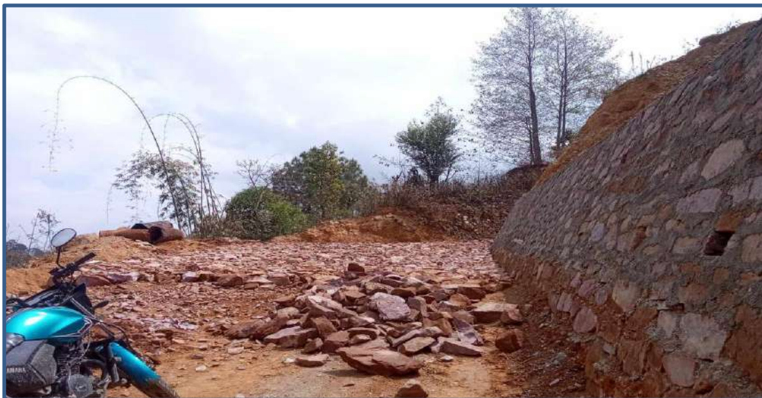
Road Soling at Box Cutting Section Salyan
