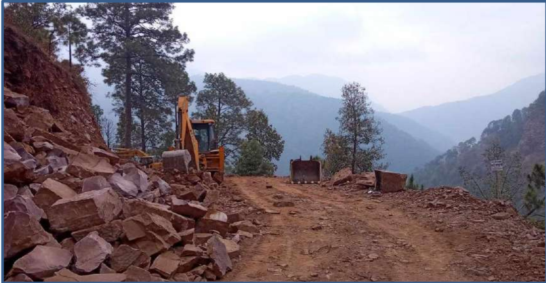
road widening and grade cutting
