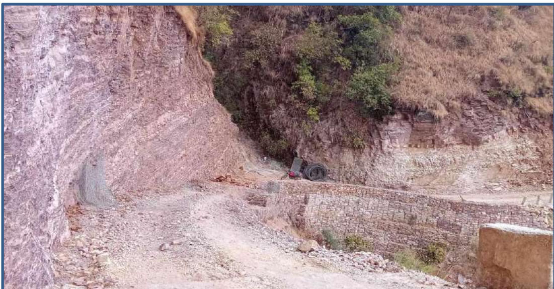
Gabion works at Vir Section
