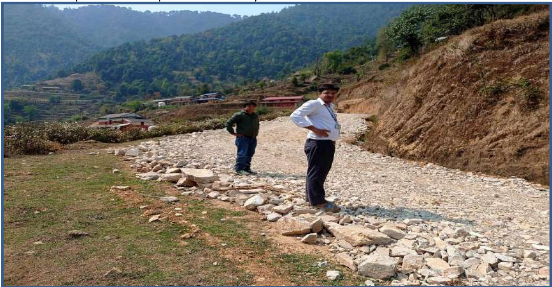
Preparation for Gravel laying at Sukhaura
