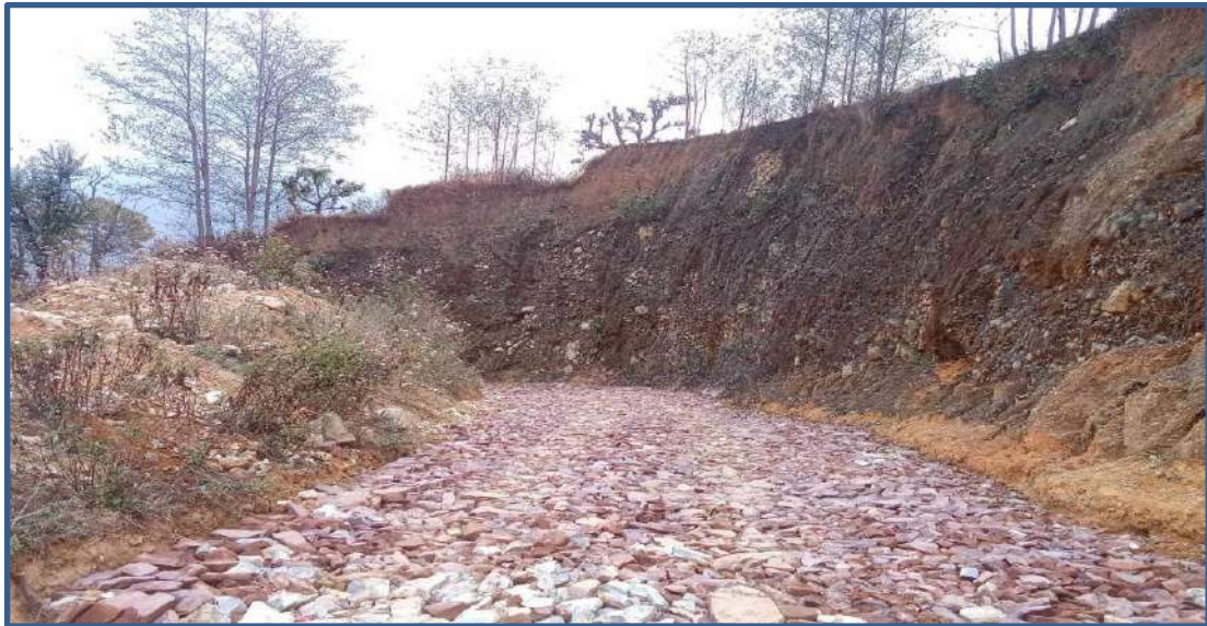
stone soling at box cutting
