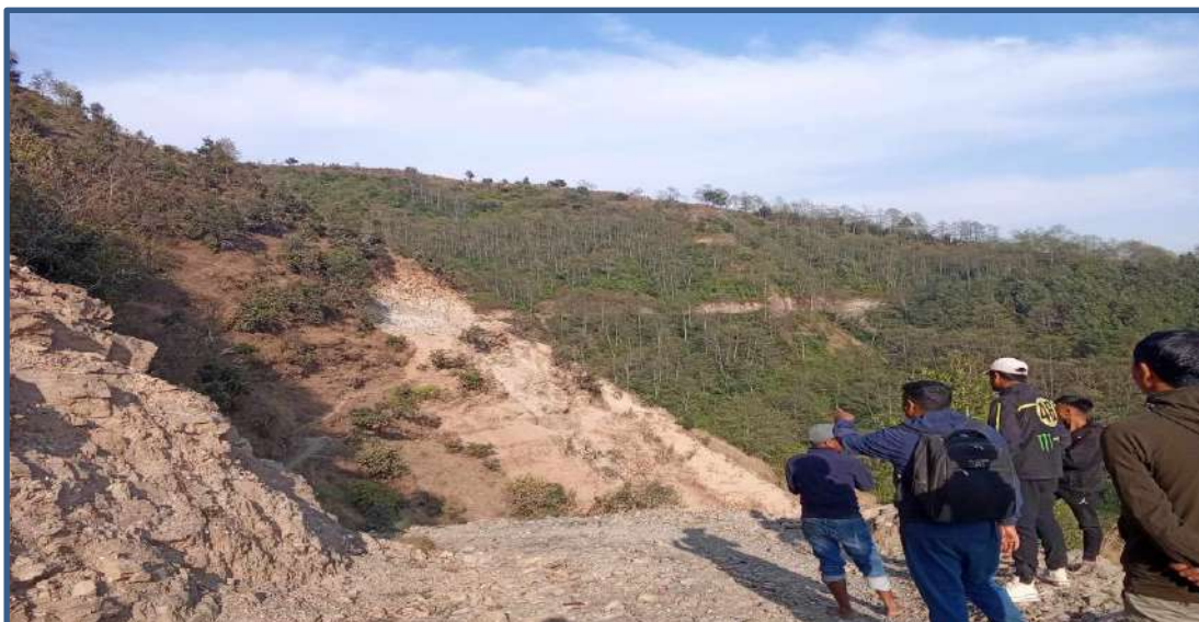
Site Inspection by Rural Municipality Team (Daduwa-Thaple Road section)
