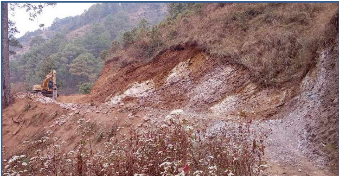
road widening and grade cutting
