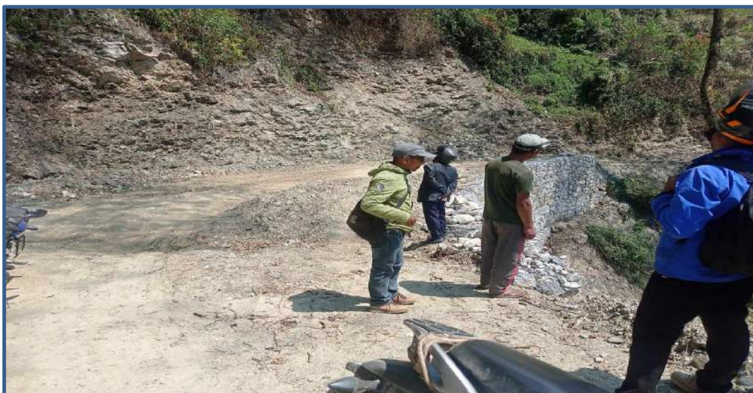
Gabion works at Lugrung-Jhule road section
