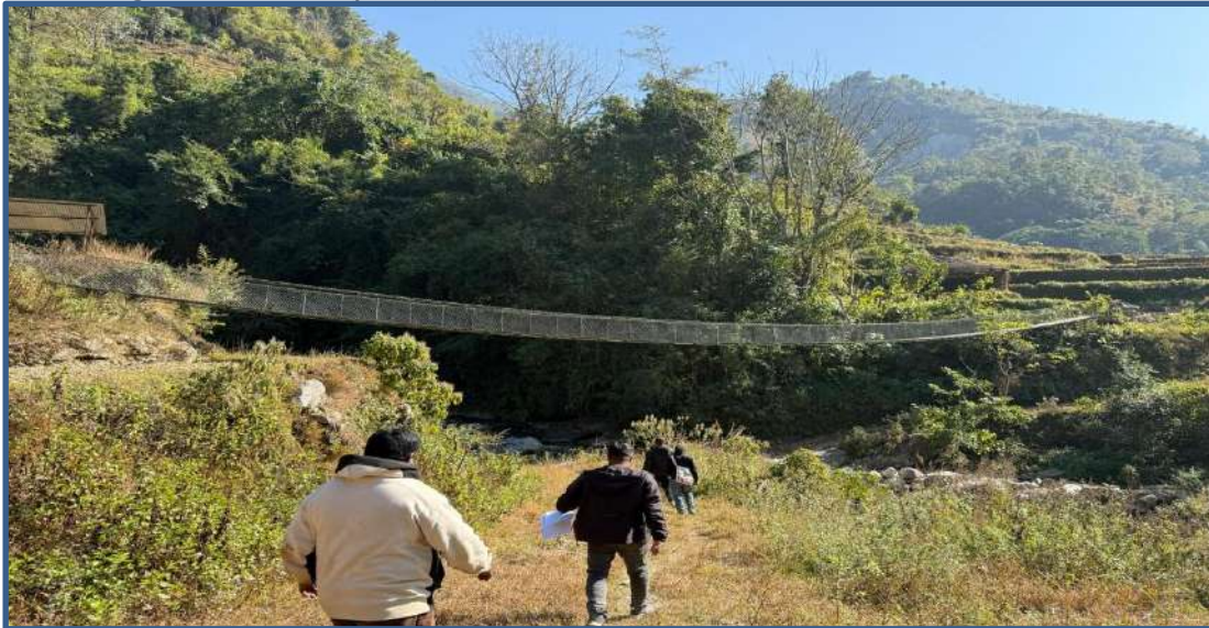
site inspection by municipality's official
