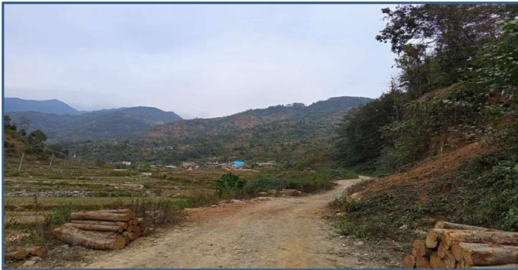
Site preparation for construction
