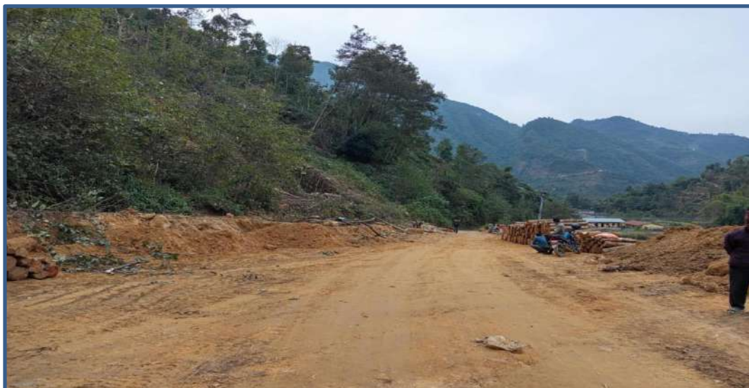
Road Widening at Sudala-Ghatta Section
