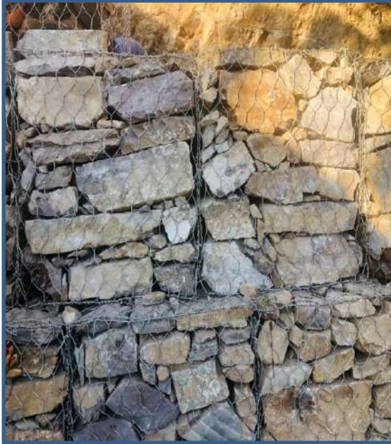
Gabion Works and Landslide clearance
