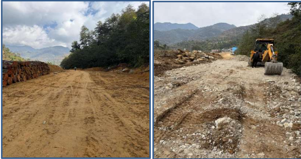
Sub-grade preparation and sub-base spreading
