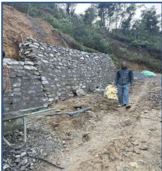
chapa cheda masonry wall and foundation
