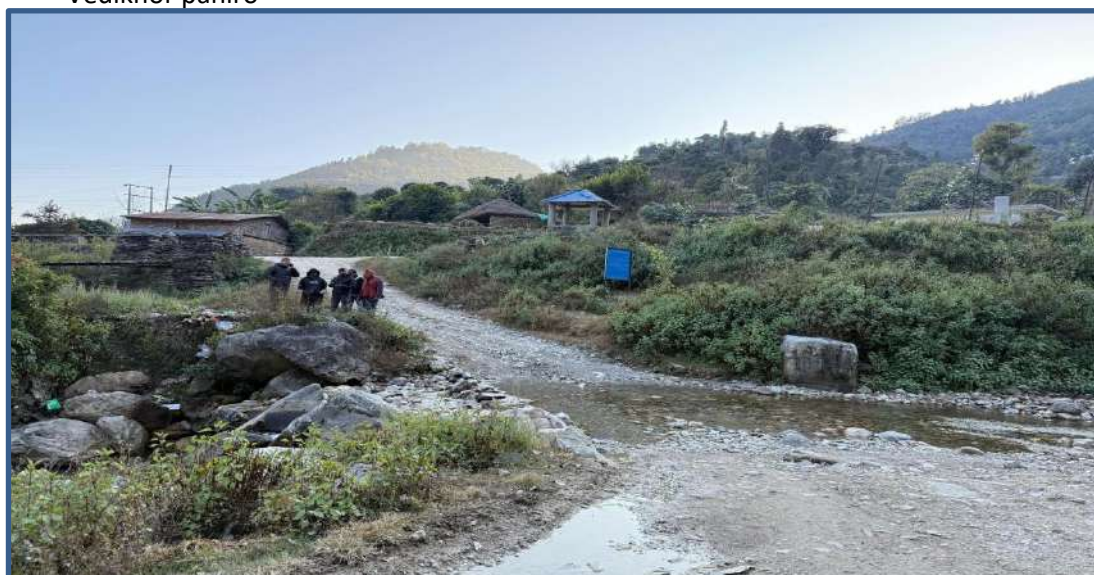
Site inspection for Thulosanghughat Motorable culvert
