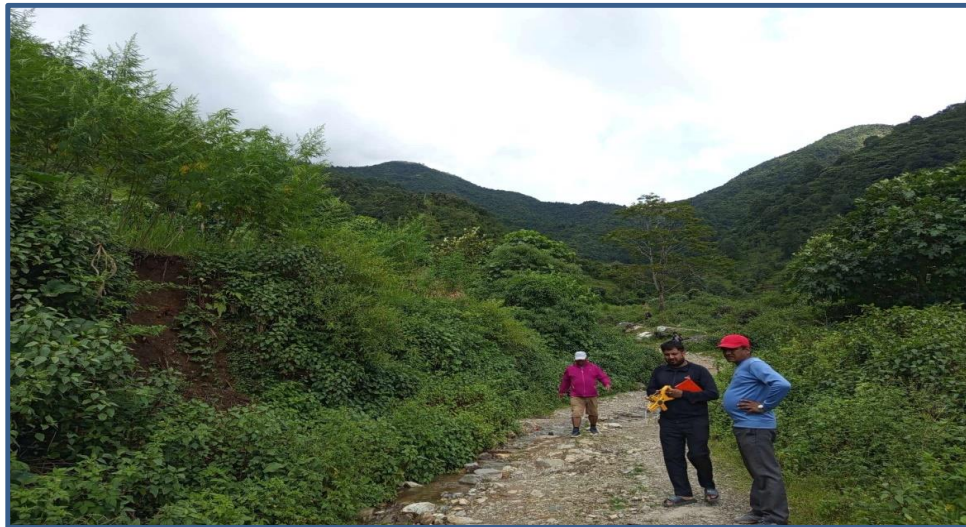
Survey for PCC Road at Barakot Phedikhola
