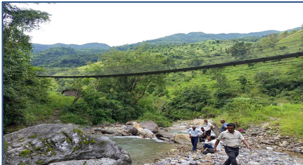
Survey for Motorable Culvert Construction
