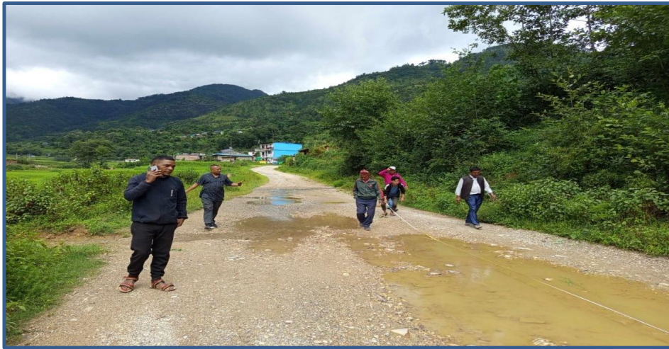
Inspection at Sudala-Ghatta Road Section
