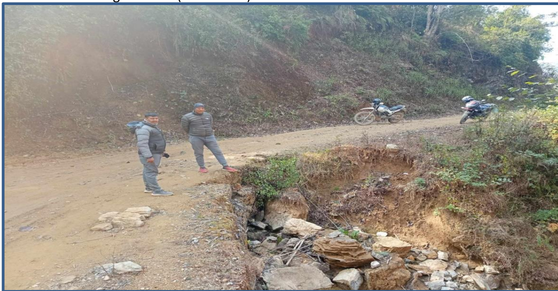
Site Inspection for Culvert Construction at Sapaude Kholsa
