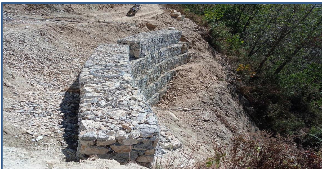
Gabion works at Jhule Section
