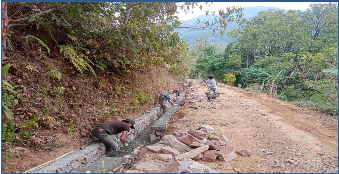
Stone masonry Drain Construction at Kudahara Section
