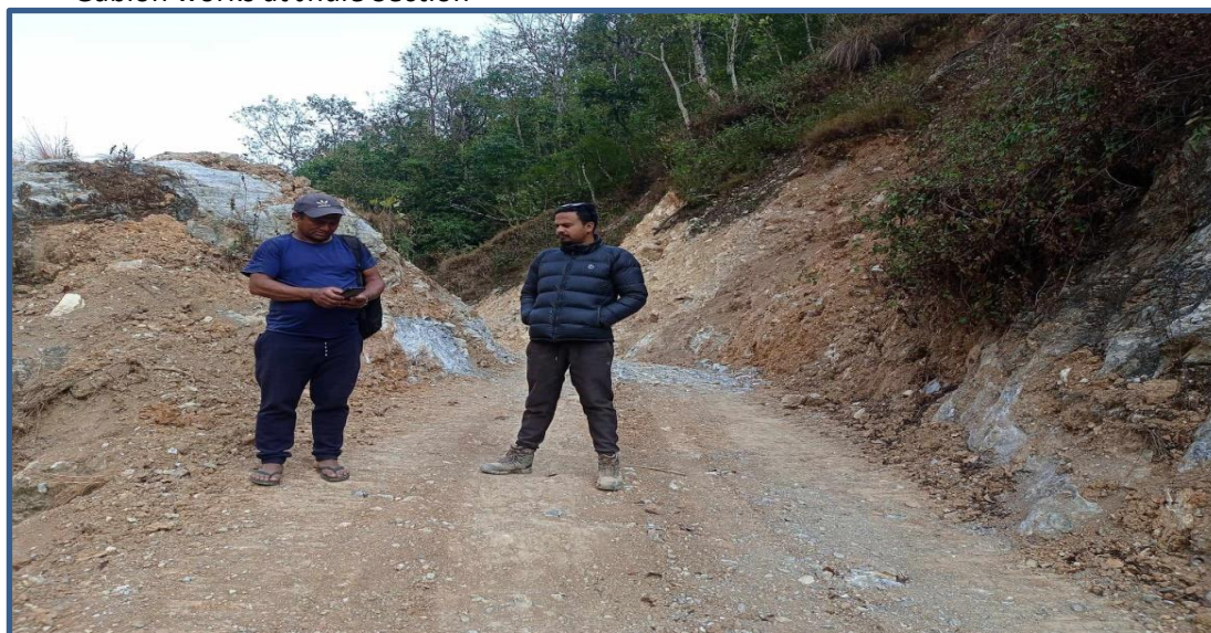
Grade Cutting works at Timureghat Section
