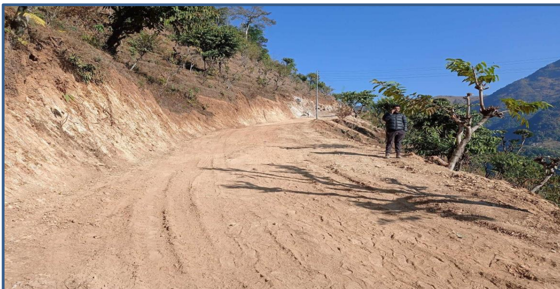
Sub-grade Prepration for Chapa-Urleni Concrete road slab
