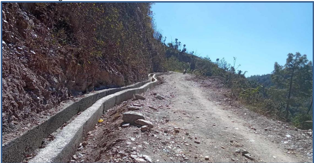
Side drain at Sakneri Difficult Section
