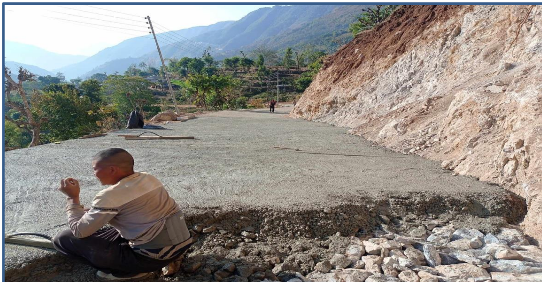
PCC Works Carried out
