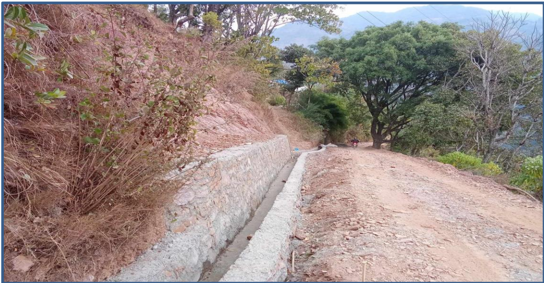
Breast Wall and Drain at Kudahara Section
