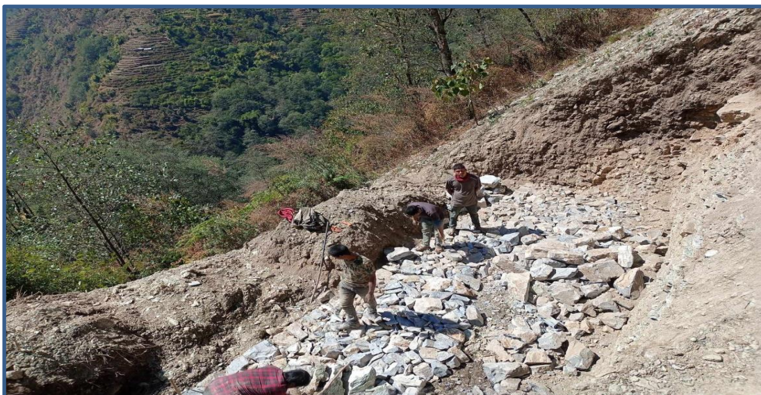
Gabion Works at Jhule-Lugrung Road section
