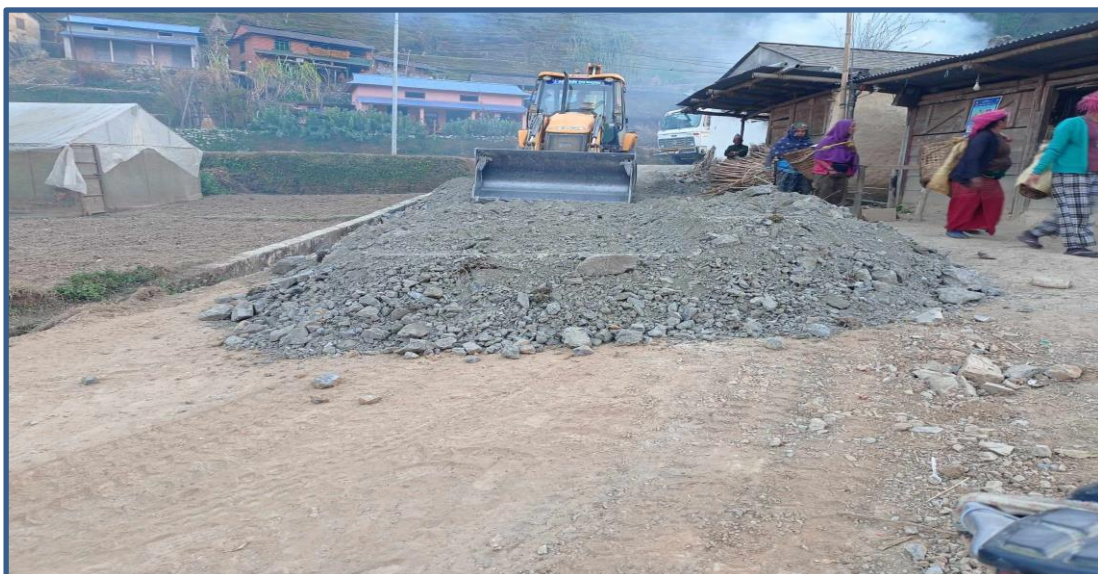
Gravelling works Started at Okhreni Village
