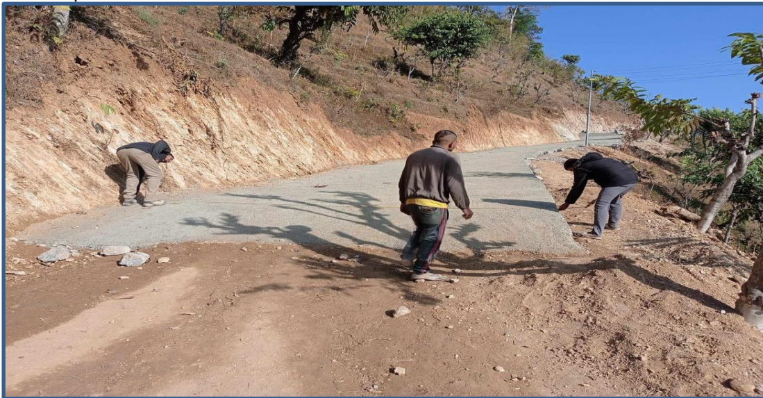
measurement of Chapa-Urleri Concrete Road Section
