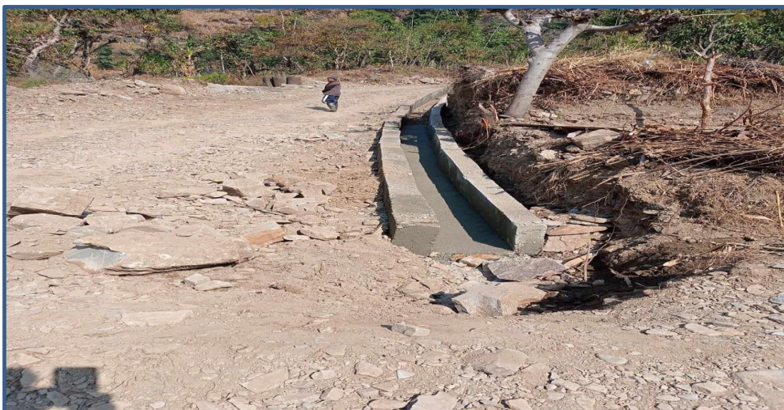
Drain at Nayabazar Road Section
