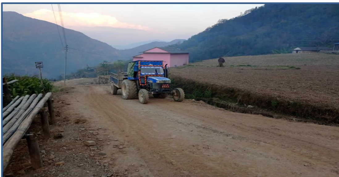
Gravelling Works Started
