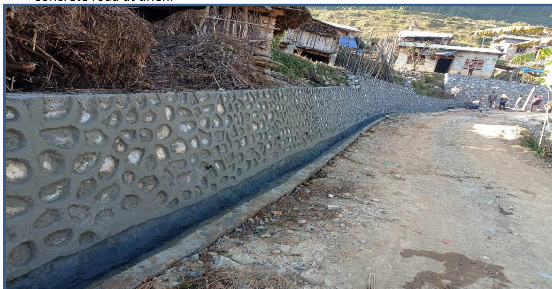
Breast wall and side drain at Okhreni Road Section
