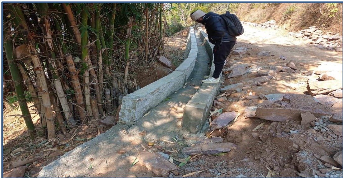
Irrigation Drain at filling side (over Retaining wall)
