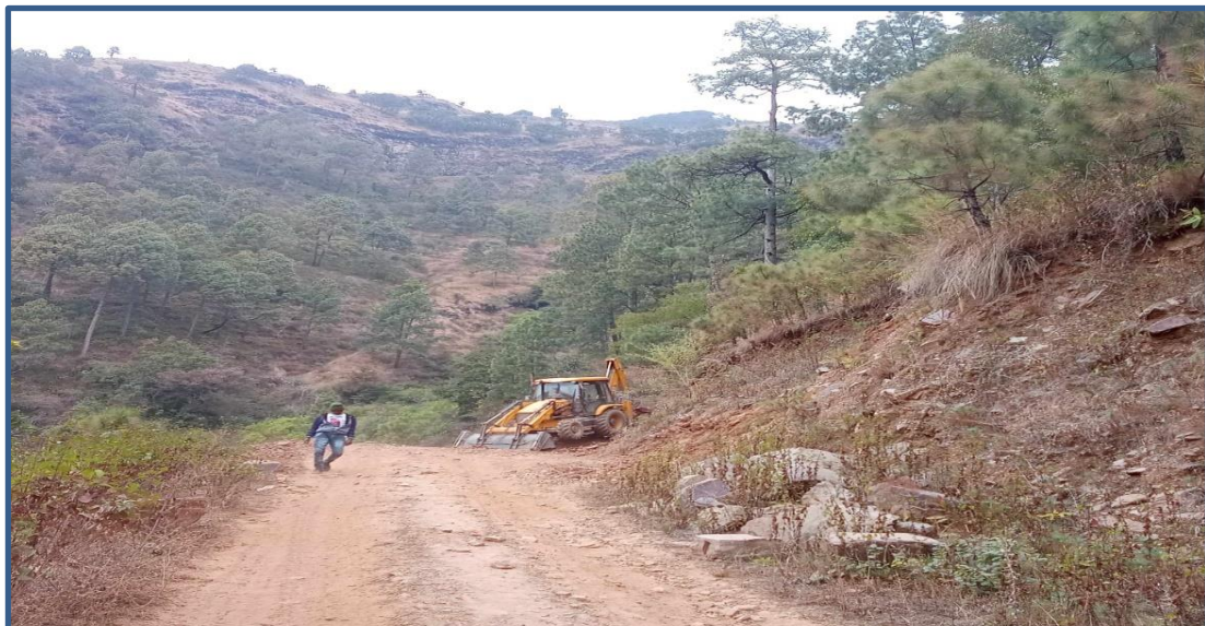
Road cutting at Vir Section
