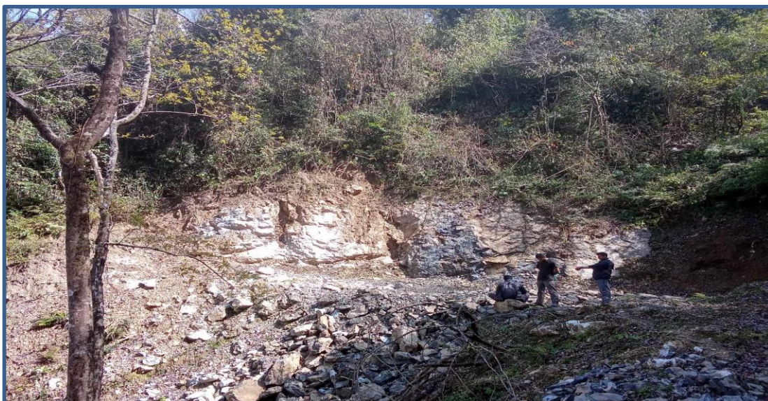
Site Inspection by Rural Municipality Officials and contractor towards Tangram site
