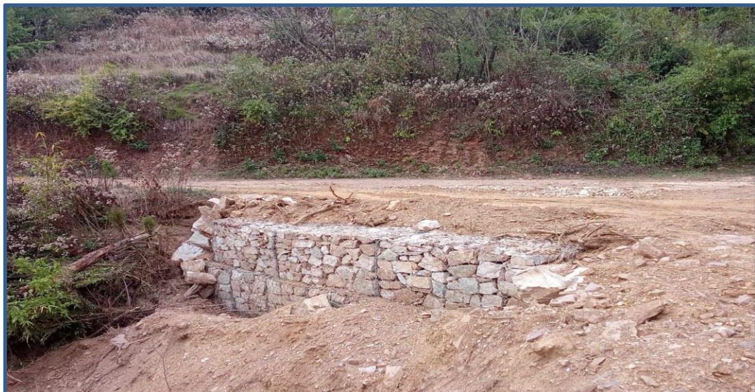
Gabion works at salyan sapaude
