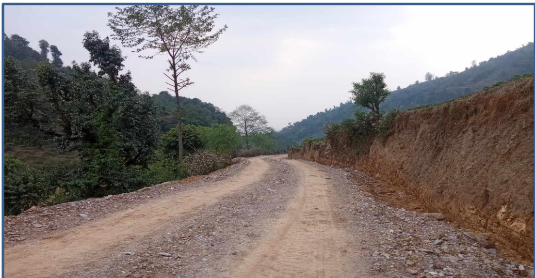
Gravel works at Vitriban road section
