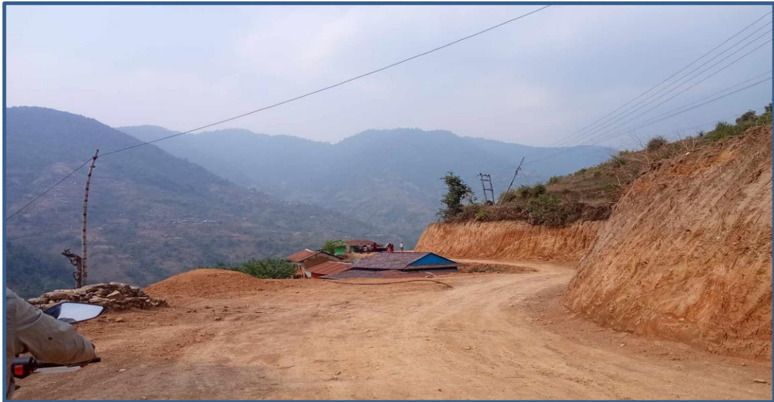
road widening at tite pakha
