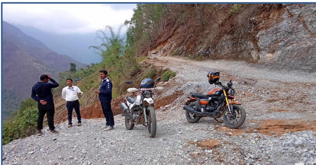
Nayabazar-Gyanodaya road section
