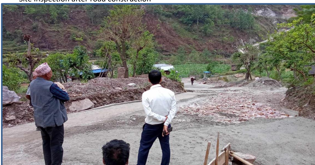
site supervision during construction
