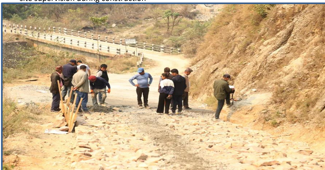
Site Inspection during construction by RM Officials
