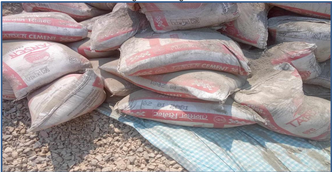
cement used at Healthdesk to Hugdikhola Bridge Road PCC
