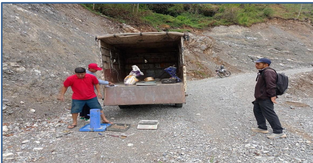
Gravelling works check at Chitrethar-Solthapa Junction
