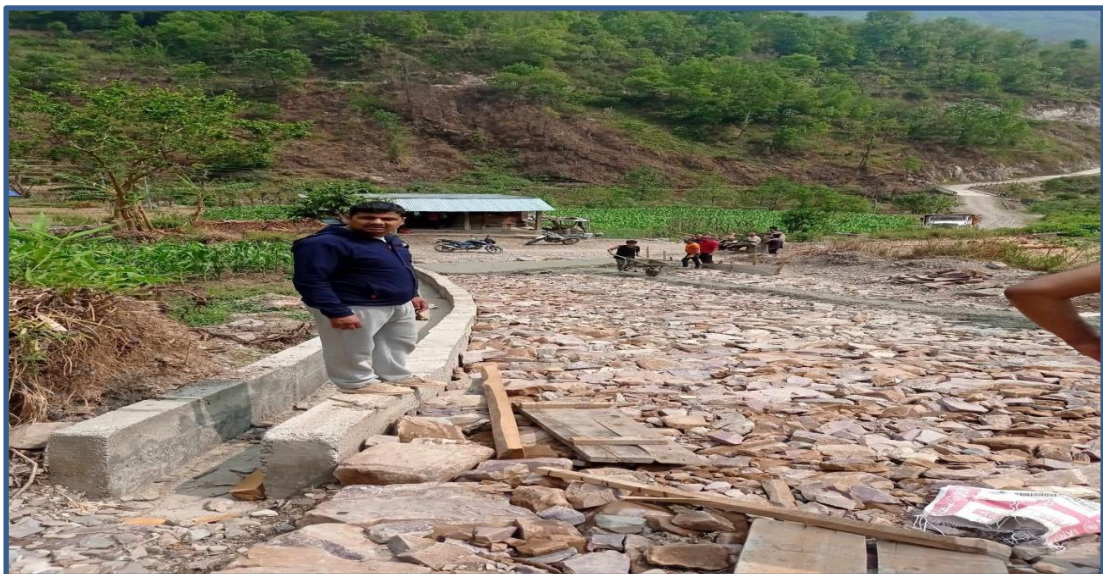
road soling for PCC road at nayabazar
