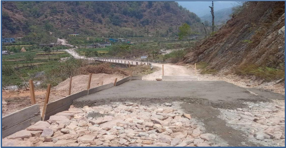
PCC Works at Healthdesk to Hugdikhola Bridge
