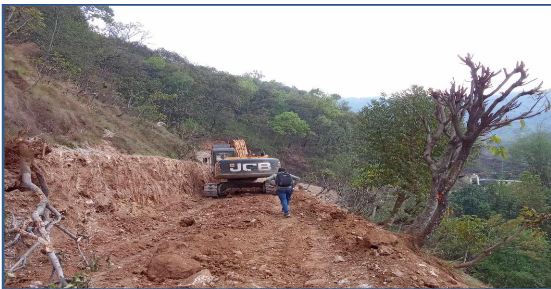
Grade down at Ligdi
