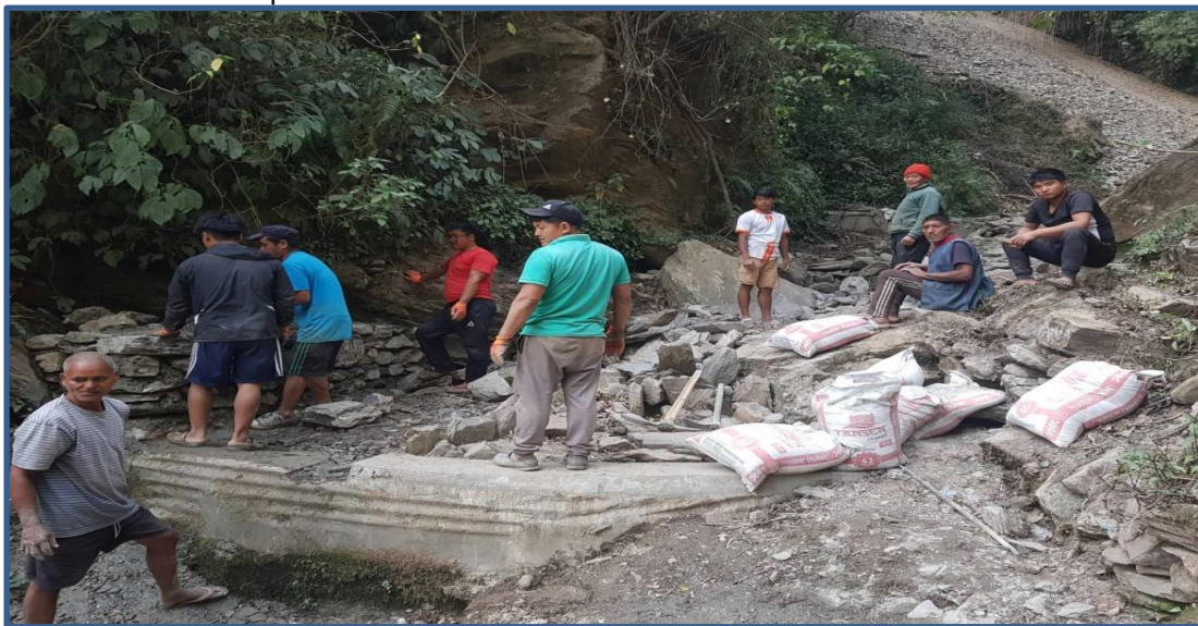
khapa muhan protection works
