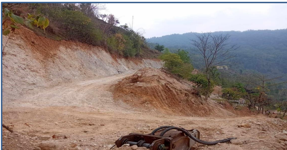
Site Inspection by Rural Municipality Officials (Ligdi Road section)
