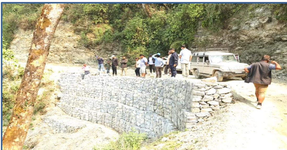
Gabion works inspection by Supervision Committee(Jhule-Lugrung Road Section)
