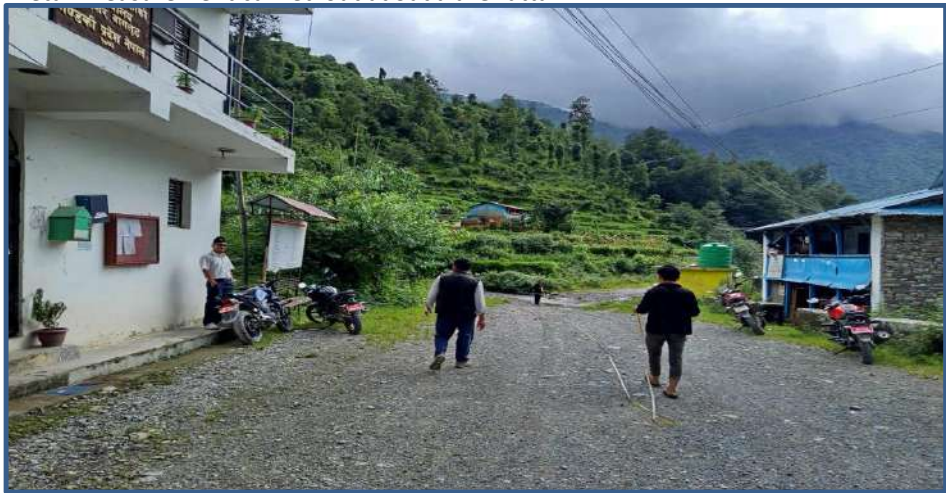
Inspection & Detail Survey at Municipal Office area
