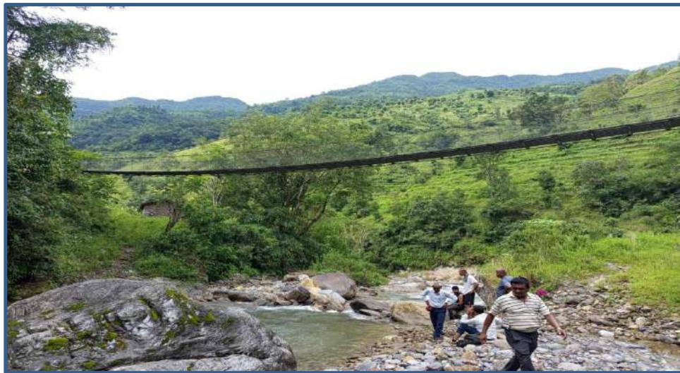
Survey for Motorable Culvert Construction
