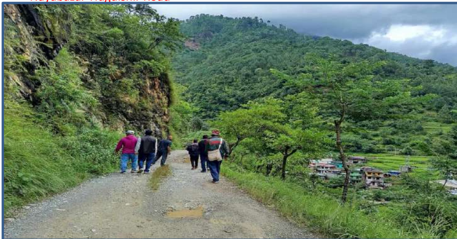
Survey at Nayabazar Difficult Road Area
