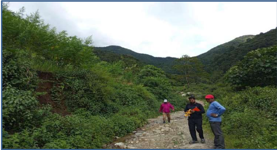
Survey for PCC Road at Barakot Phedikhola
