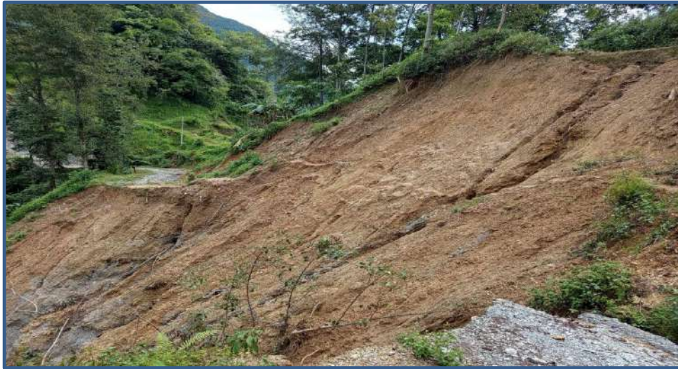
Condition of Chapa-Neta Road section (Dhullubaskot) due to huge landslide
